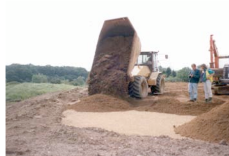
Hydrema Dump Truck placing rootzone
