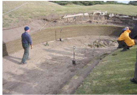
Reconstruction of a revetted links bunker: Cottage Bunker, Old Course, St Andrews
