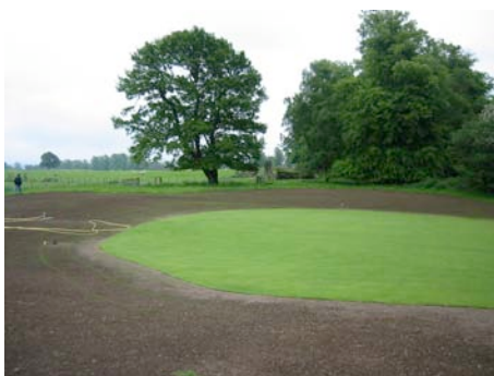
Original greens turf re-laid on new USGA green construction. Dalmahoy, Edinburgh
