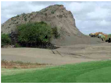
Oversized topsoil heap – potential problems with soil structure – and health and safety!
