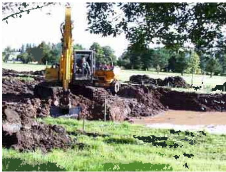
Pond excavation, Auchterarder Golf Club, Perth and Kinross
