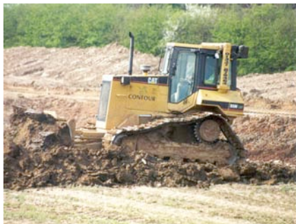
Topsoil being stripped by Caterpillar D5 dozer
