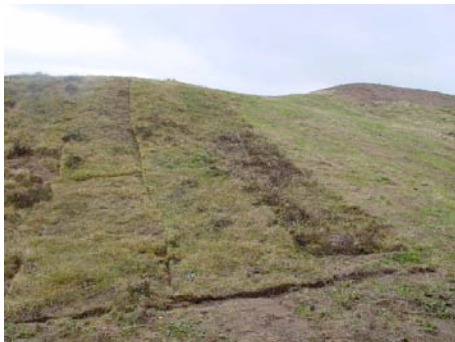
Heather turves stripped on-site and re-used on new mound. Dundonald Links, Ayrshire
