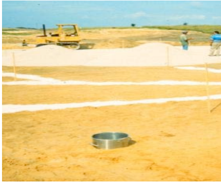
Lysimeter installed in green sub-base. (Photo Turf-Tec International, Florida)
