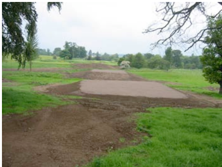
New tee platforms showing USGA rootzone, with topsoiled surrounds. Dalmahoy, Edinburgh
