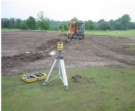
Drainage trench invert being controlled by laser levelling
