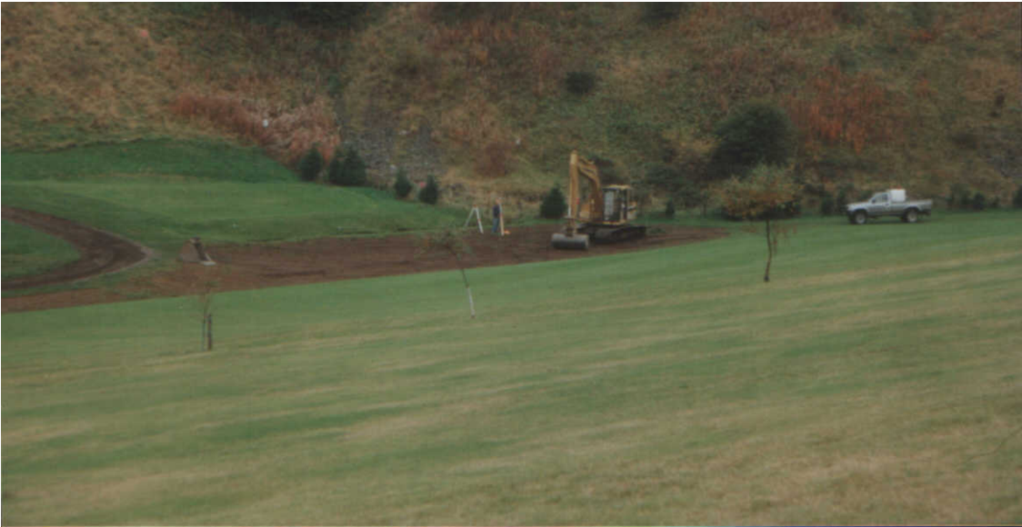
Pond during construction
